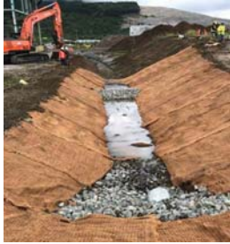
Pond 9 flume installation
