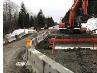
Bish Forest Service Road (FSR) culvert replacement
