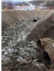
Temporary repair to Haul Road sink hole
