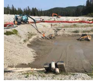
LNG plant site storm water pond cleanout
