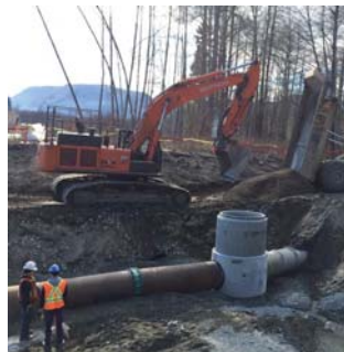
Installation of manhole
