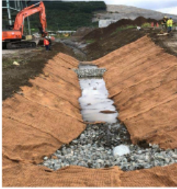
Pond 9 flume Installation
