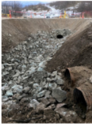
Temporary repair to Haul Road sink hole
