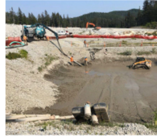
LNG plant site storm water pond cleanout
