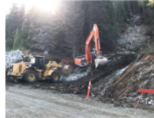
Bish FSR landslide repairs
