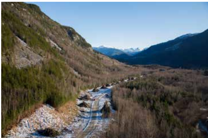
Pacific Trail Pipeline right-of-way
